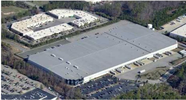
EMC's new data center in Durham, NC
